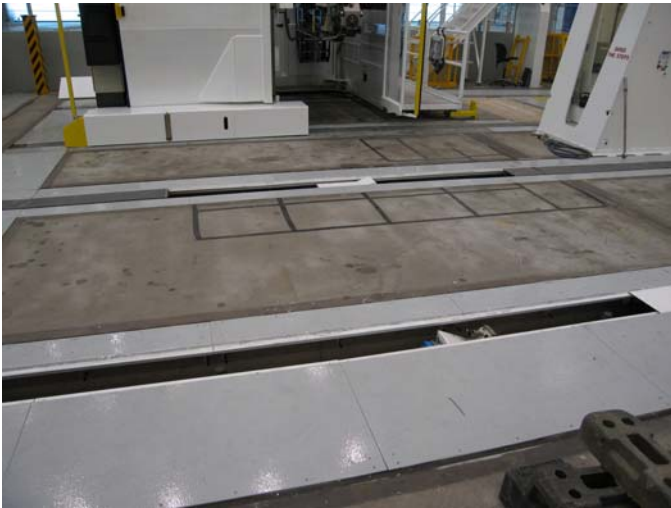
Figure 3 – Flush Factory Floor – Machine Absent, Infill Boards Removed
